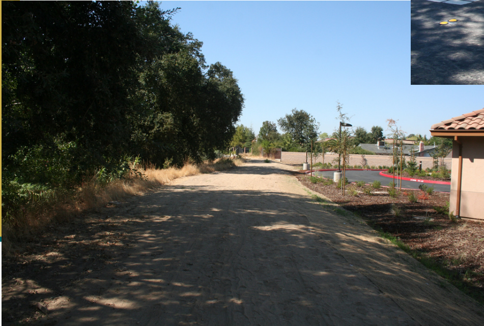
SEWER MAINTENANCE ROAD BETWEEN EICH AND ROCKY RIDGE
